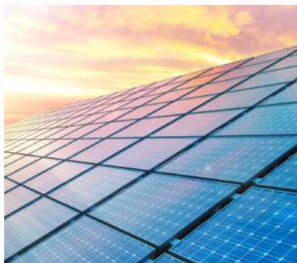
Solar Array Testing
